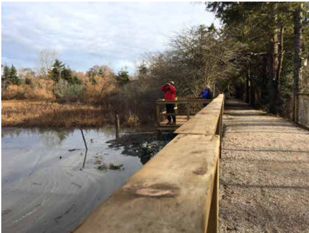
North Dyke fencing and deck
