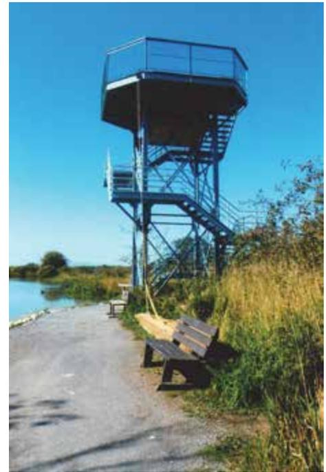
*The blue metal tower was built in 1981 in the West Field to replace the wooden tower. The metal was salvaged from scaffolding used in the construction of the atriums of Lansdowne Shopping Center in Richmond.*
