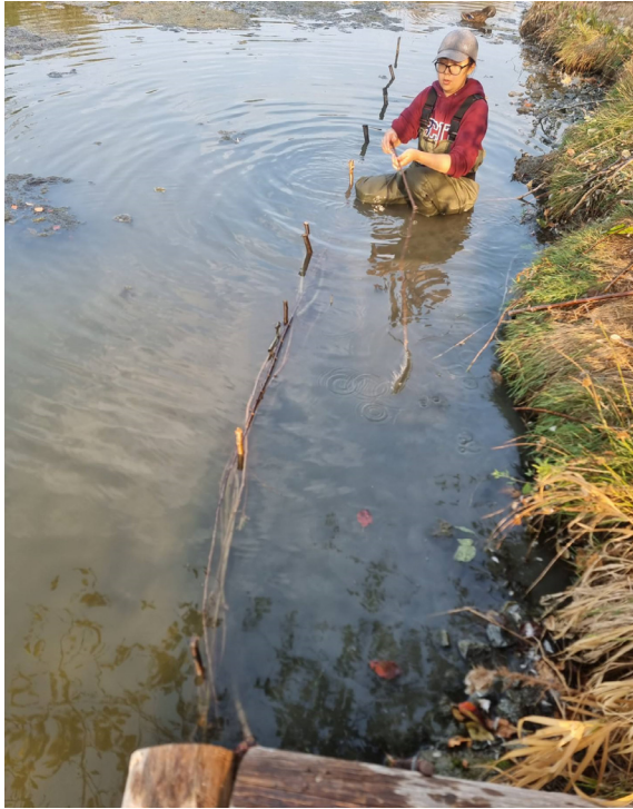
Photos of the shoreline enhancement project along the Auger Trail, using “soft engineering” methods such the wattle fencing being woven by Marissa Sasaki (above) and backfilling of areas shaped by sandbags of gravel and topsoil. Photos: Evan Gogal
