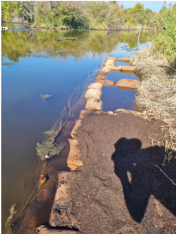
Photos of the shoreline enhancement project along the Auger Trail, using “soft engineering” methods such the wattle fencing being woven by Marissa Sasaki (above) and backfilling of areas shaped by sandbags of gravel and topsoil. Photos: Evan Gogal
